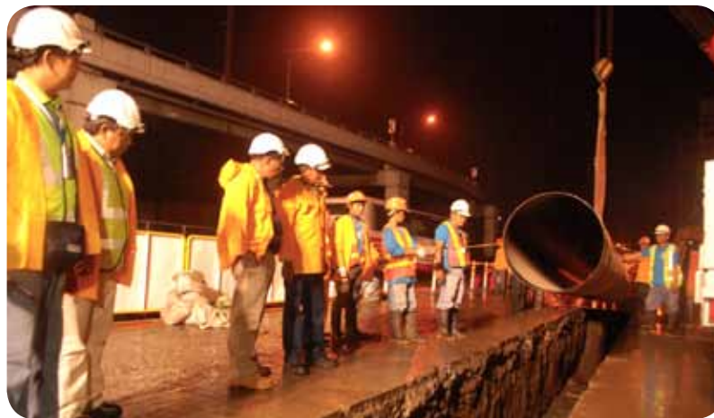
Manila Water has installed 441 linear meters for its pipe-laying operations
